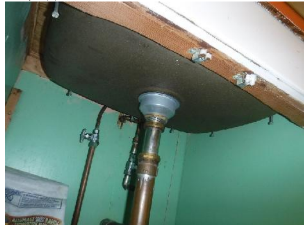
Photo 4 Description: Acoustic sink insulation – black/gold Location: Classroom 6 Asbestos: 20% chrysotile Sample(s): 30015-10
