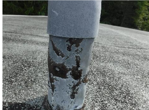
Photo 2 Description: Mastic (Black) Location: Roof Asbestos: 9% chrysotile Sample(s): 39956-11b
