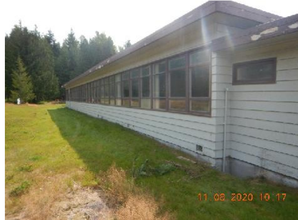
Photo 6 Description: Window putty/caulking - off-white
