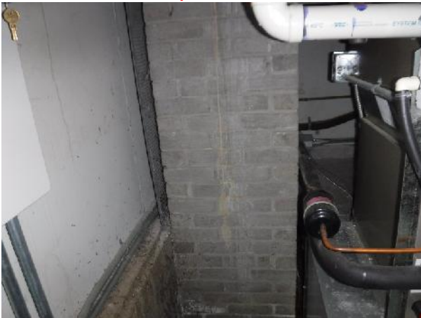
Photo 5 Description: Brick and mortar Location: Furnace Room Asbestos: Suspect
