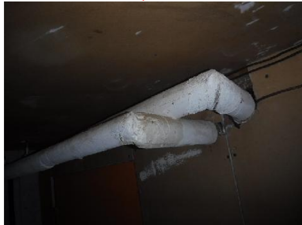
Photo 6 Description: Textile wrapped fibreglass insulation Location: Maintenance Shop Asbestos: Suspect
