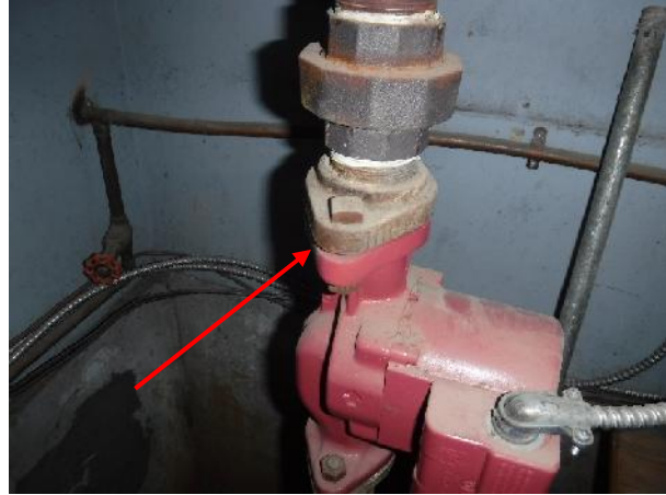
Photo 6 Description: Gasket Location: Boiler Room Asbestos: Suspect
