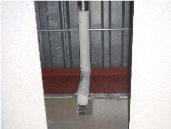
Photo 5 Description: Pipe run insulation Location: Room 304 Asbestos: Suspect
