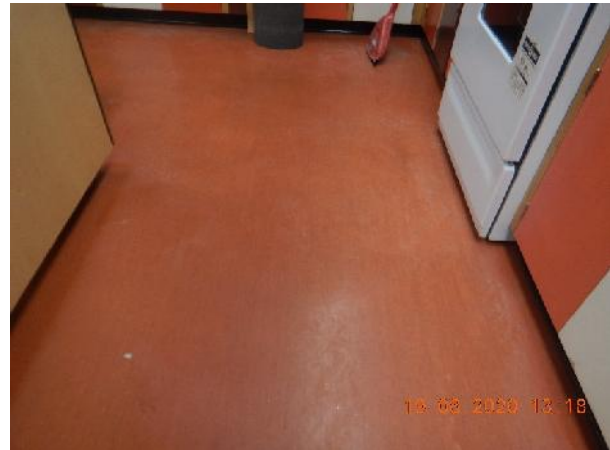
Photo 2 Description: Sheet flooring 3 – red Location: Kitchen off Gym Asbestos: 2.4% chrysotile Sample(s): 30013-2
