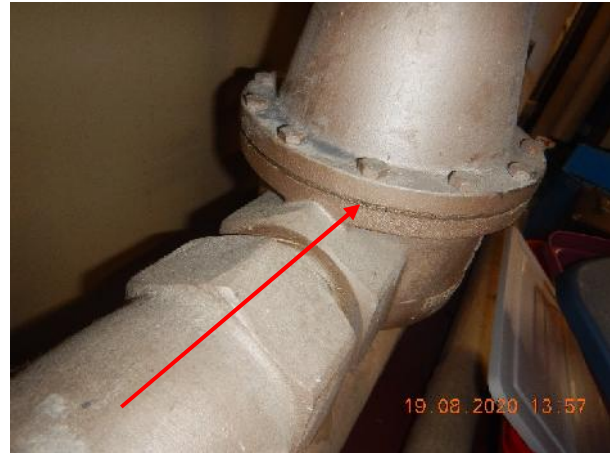
Photo 6 Description: Gasket Location: Mezzanine Book Room Asbestos: Suspect
