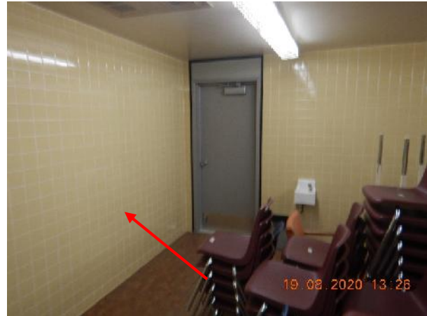
Photo 6 Description: 6"x6" yellow ceramic tile grout Location: Girls Change Room Off Gym Asbestos: Suspect
