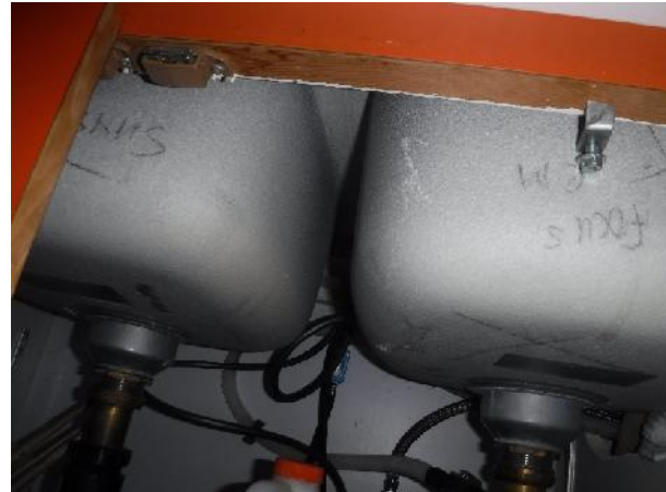
Photo 6 Description: Acoustic sink insulation – white Location: Room 305 Asbestos: Suspect
