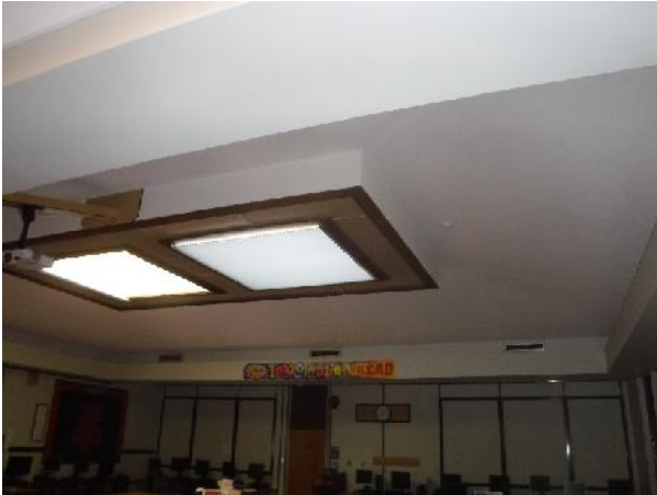
Photo 5 Description: Texture coat Location: Room 333 Learning Commons Asbestos: Suspect
