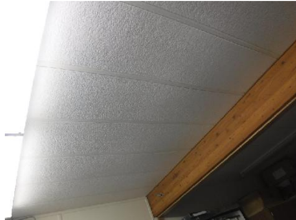
Photo 8 Description: Trailer type ceiling panel Location: Portable Trailer Asbestos: Suspect
