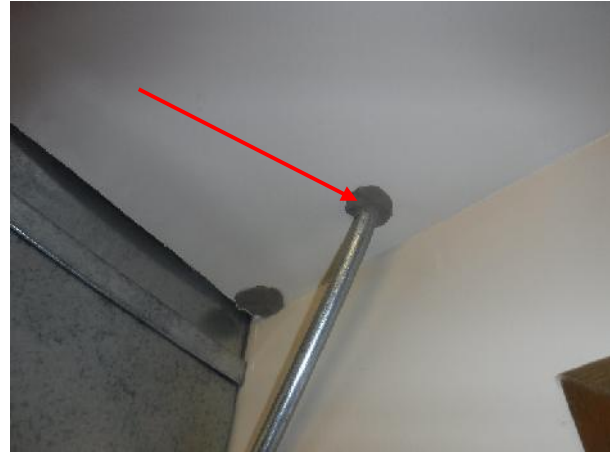
Photo 10 Description: Caulking type 2 – grey around electrical penetration Location: Vault Asbestos: Suspect
