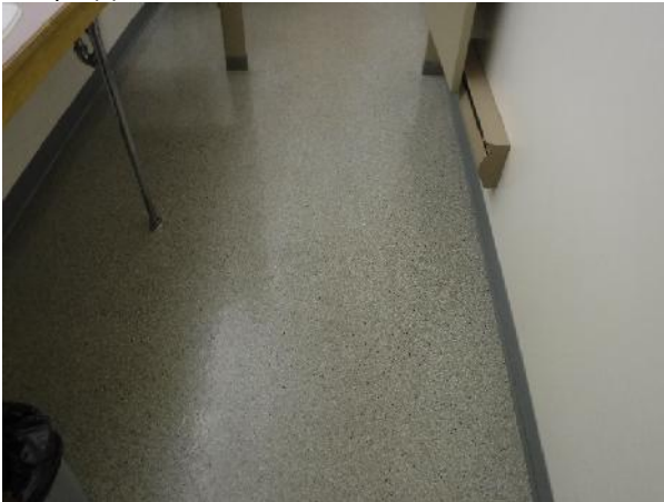
Photo 3 Description: Sheet flooring 1 – grey white black speckles Location: Female Washroom Asbestos: Suspect
