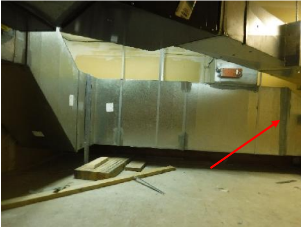
Photo 9 Description: Caulking type 1 – grey Location: Mezzanine Above Copy Room Asbestos: Suspect
