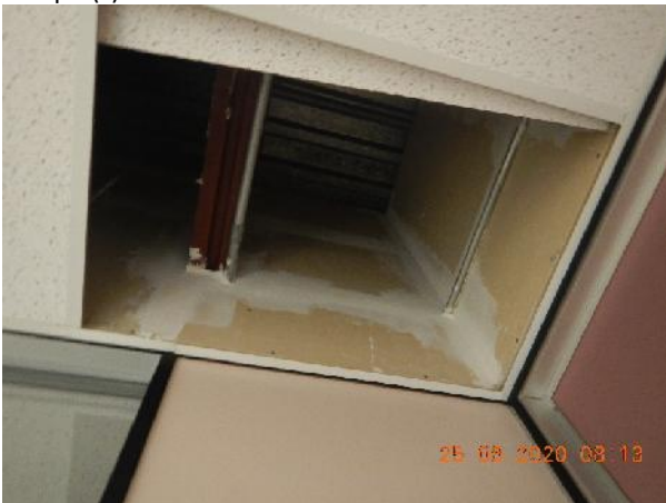
Photo 3 Description: Drywall joint compound Location: Room 310 Asbestos: 1.5%chrysotile Sample(s): 31788-6b
