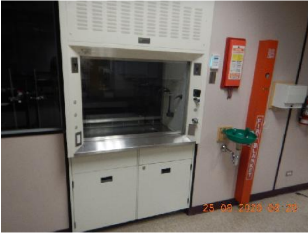
Photo 25 Description: Fume hood cement board Location: Room 320 Asbestos: Suspect
