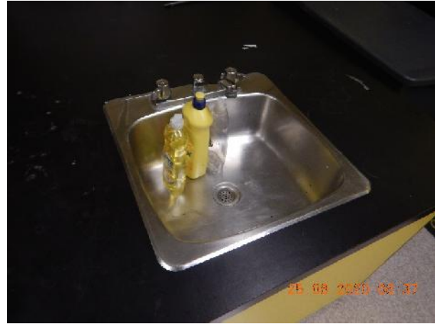
Photo 26 Description: Counter tops Location: Room 340 Asbestos: Suspect
