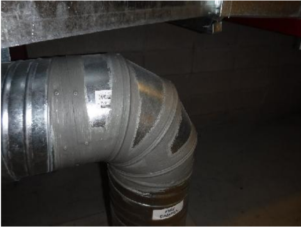
Photo 17 Description: Caulking – grey Location: Room 209 ducting Asbestos: Suspect
