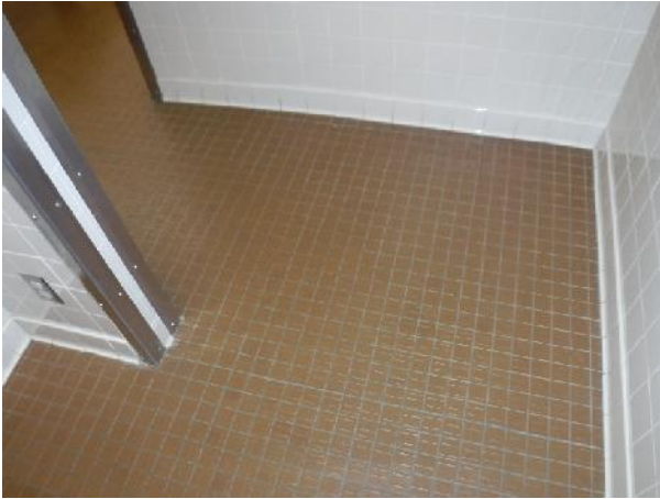
Photo 9 Description: Ceramic tile – 1"x1" brown Location: Women's Change Room Asbestos: Suspect
