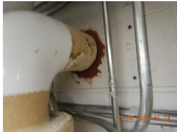
Photo 20 Description: Firestop – red Location: 645 Mezzanine Boiler Room Asbestos: Suspect
