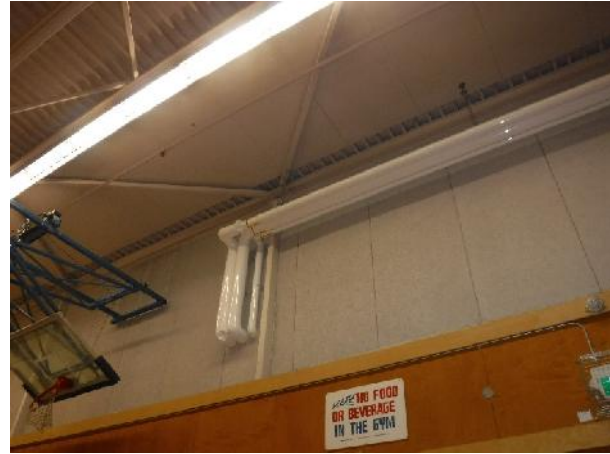
Photo 14 Description: Acoustic wall board Location: Gym Asbestos: Suspect
