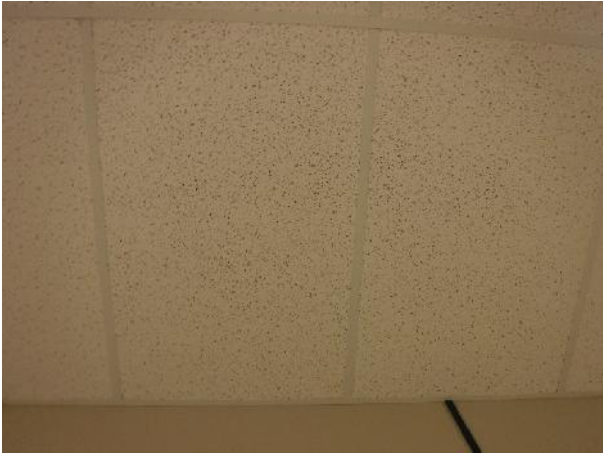
Photo 5 Description: Acoustic ceiling tile 2 – random fissure large pinhole Location: Room 205 Asbestos: Suspect
