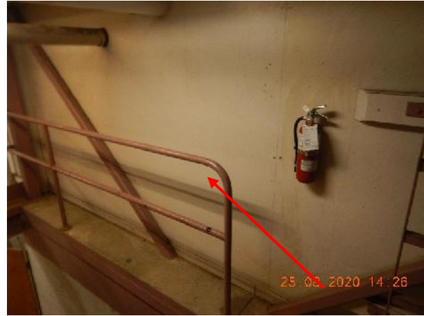
Photo 22 Description: Cement board Location: Room 645 Stairwell Asbestos: Suspect
