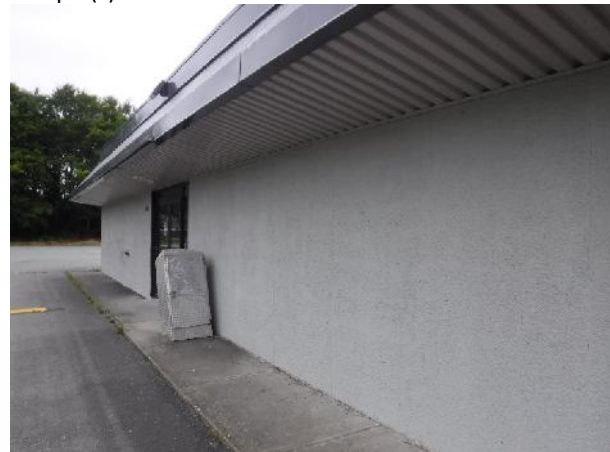
Photo 4 Description: Stucco Location: Exterior Asbestos: Suspect
