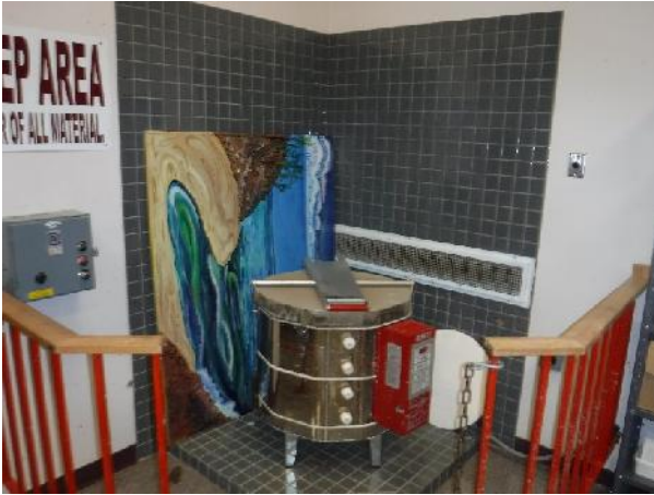
Photo 13 Description: Ceramic tile – 4”x4” dark grey Location: Room 675 Asbestos: Suspect
