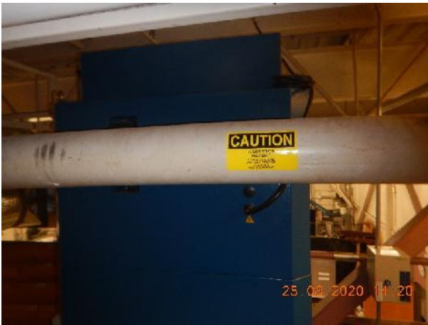
Photo 23 Description: Cement pipe Location: Room 645 Mezzanine Asbestos: Confirmed (labelled on site)
