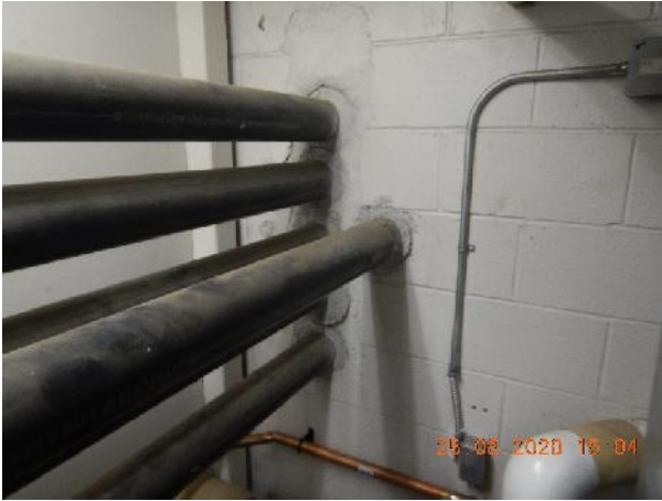
Photo 21 Description: Parging – grey Location: 645 Mezzanine Boiler Room Asbestos: Suspect
