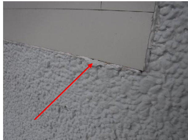
Photo 16 Description: Caulking – grey Location: Exterior siding Asbestos: Suspect
