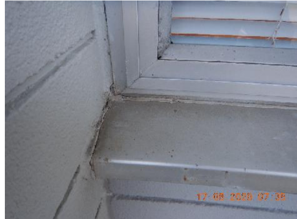
Photo 2 Description: Caulking 3 – Grey Location: Exterior Asbestos: 1.3% Chrysotile Sample(s): 30007-27
