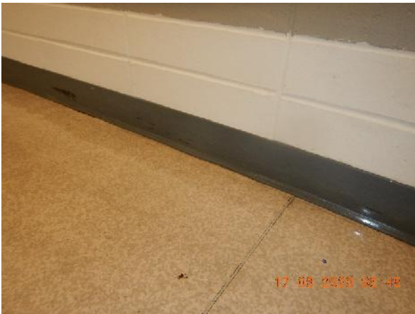
Photo 13 Description: Baseboard adhesive Location: Room 101 Asbestos: Suspect
