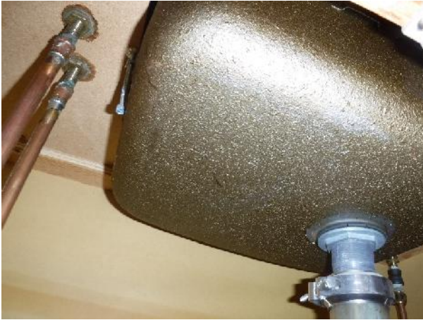
Photo 7 Description: Mastic 3 – Black/Silver on sink Location: Room 231 Asbestos: 1.3% Chrysotile Sample(s): 30007-21
