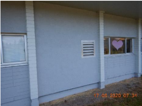
Photo 9 Description: Stucco Location: Exterior Asbestos: Suspect
