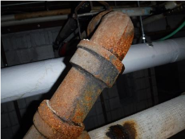
Photo 21 Description: Bell and spigot pipe gaskets Location: Crawl Space Asbestos: Suspect
