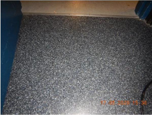
Photo 27 Description: Sheet flooring 2 – Grey and speckled pattern Location: Drama Asbestos: Suspect
