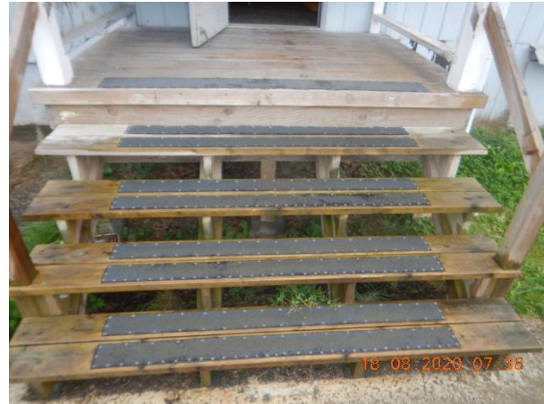
Photo 4 Description: Asphalt stair tread Location: Exterior Asbestos: Suspect
