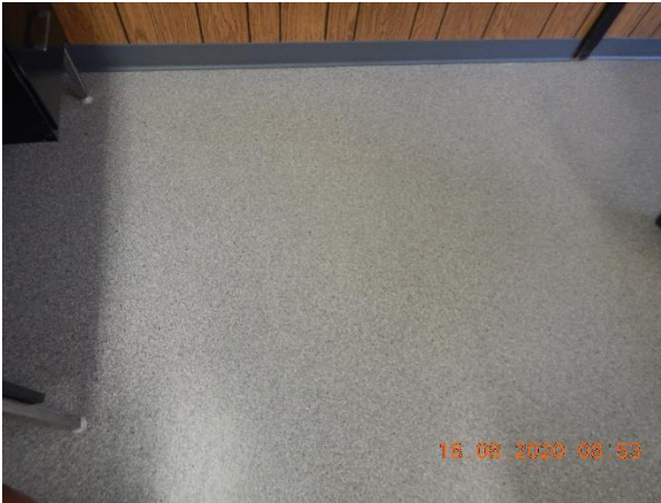
Photo 11 Description: Baseboard Adhesive Location: Room 1 Asbestos: Suspect
