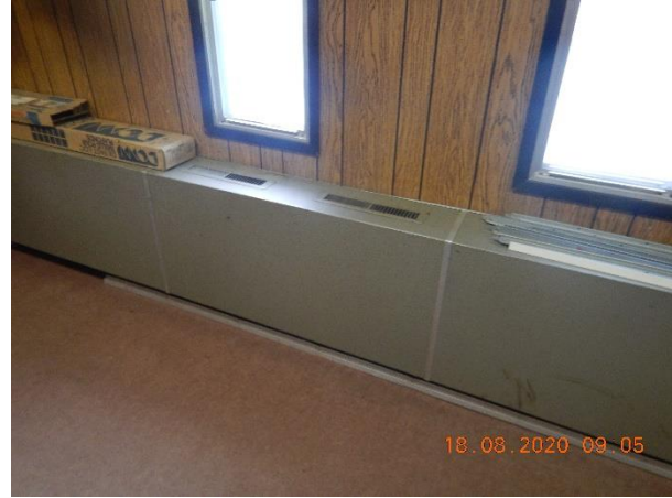
Photo 10 Description: Radiator (may contain concealed ACM insulation) Location: Room 2 Asbestos: Suspect
