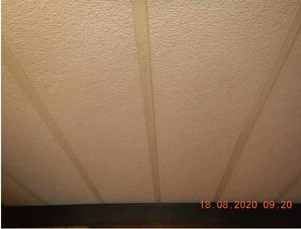
Photo 9 Description: Acoustic ceiling tile 1 – Textured Location: Room 4 Asbestos: Suspect
