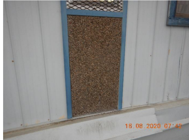
Photo 2 Description: Aggregate panel Location: Exterior Asbestos: Suspect
