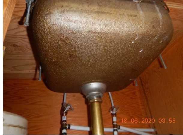
Photo 6 Description: Mastic 2 – Gold/silver Location: Room 1 Asbestos: Suspect
