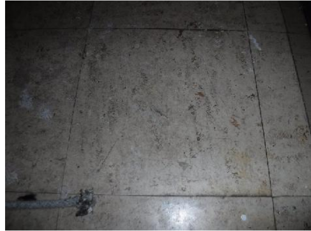
Photo 6 Description: Floor tile 3 – Beige with red and brown streaks
