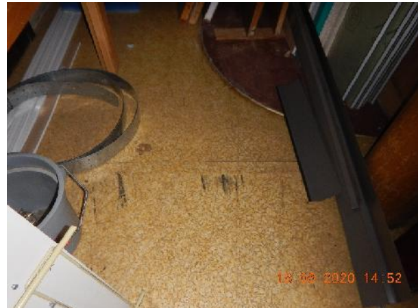
Photo 2 Description: Sheet flooring 13 – Yellow swirl Location: Storage Room I Asbestos: 20% Chrysotile Sample(s): 30008-9
