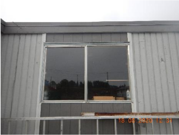
Photo 5 Description: Caulking type 1 – White/grey
