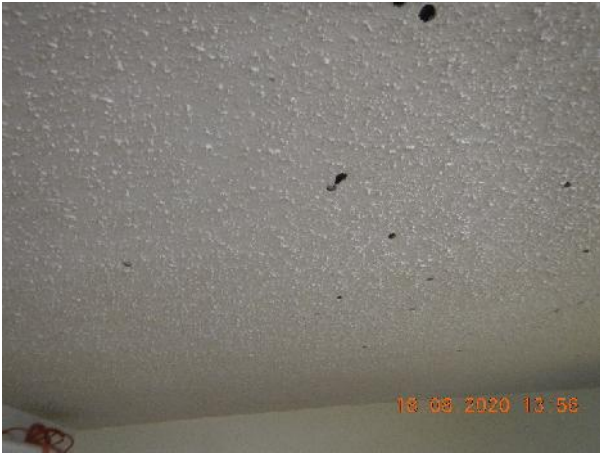
Photo 7 Description: Texture coat Location: Storage Room L Asbestos: Suspect
