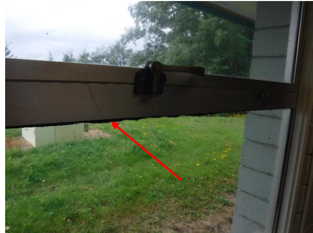
Photo 8 Description: Window mastic – Black
