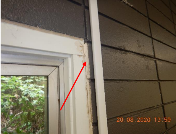
Photo 9 Description: Caulking – Off White Location: Meeting Room 1 Asbestos: Suspect
