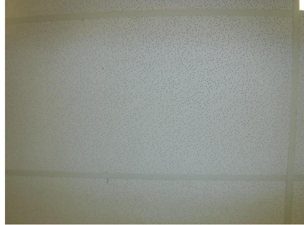
Photo 6 Description: Acoustic ceiling tile type 1 – Small and large pinhole
