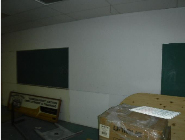
Photo 5 Description: Drywall with joint compound
