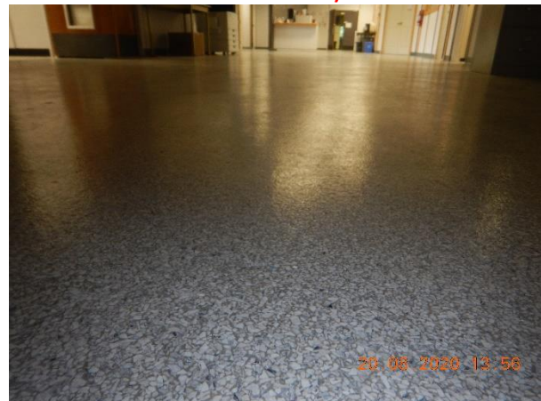
Photo 4 Description: Sheet flooring 2 – Grey and black Location: Main Hallway Asbestos: Suspect
