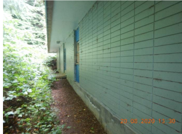
Photo 2 Description: Concrete block Location: Exterior Asbestos: Suspect (may contain vermiculite)
