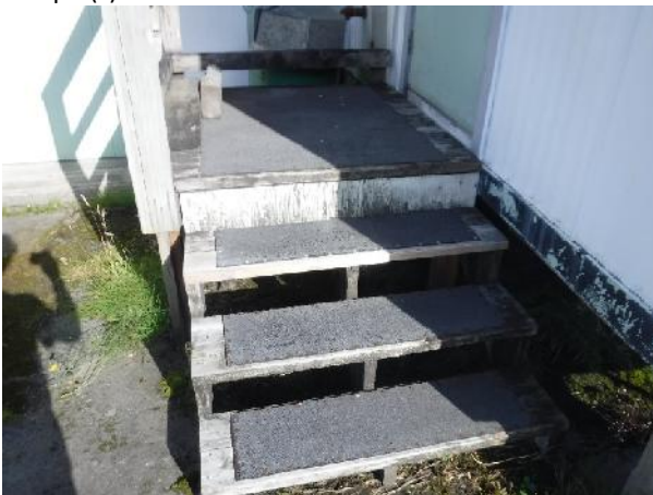
Photo 3 Description: Asphalt stair tread Location: Exterior stairs Asbestos: Suspect
