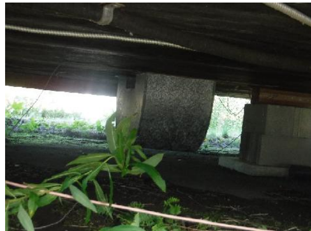
Photo 4 Description: Mastic – grey Location: Ductwork Beneath Trailer Asbestos: Suspect
