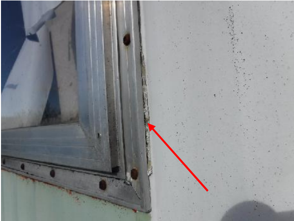
Photo 1 Description: Caulking – off white Location: Main Room Asbestos: 15% Chrysotile Sample(s): 30014-15
