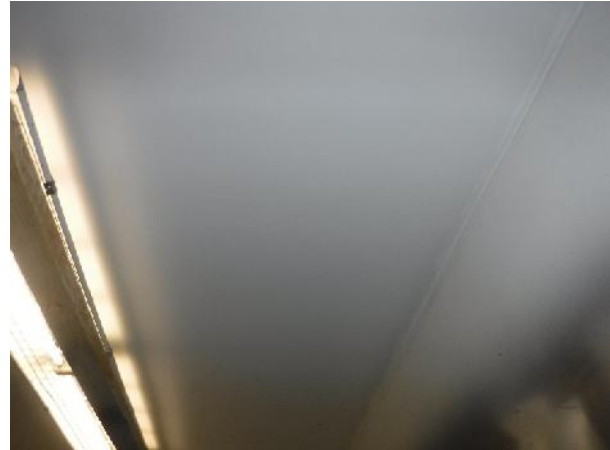
Photo 2 Description: Drywall joint compound Location: Storage Room Asbestos: Suspect
