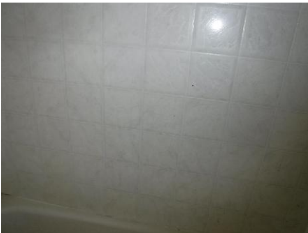
Photo 3 Description: Sheet flooring 3 – off white 9"x9" pattern Location: Bathroom Asbestos: Suspect
