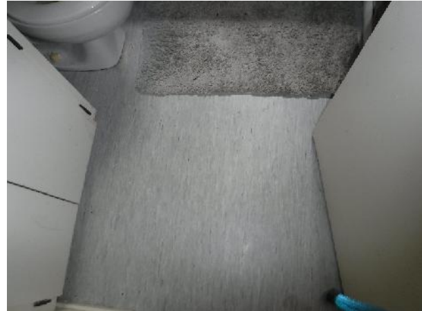
Photo 2 Description: Sheet flooring 2 – grey streaked Location: Bathroom Asbestos: Suspect
