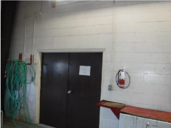
Photo 1 Description: Concrete block wall (may contain vermiculite) Location: Garage Asbestos: Suspect
