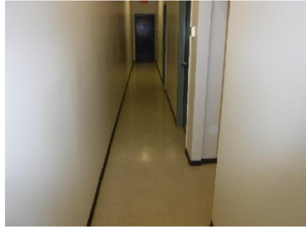
Photo 6 Description: Baseboard adhesive Location: Entryway Asbestos: Suspect
