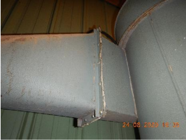
Photo 5 Description: Gasket Location: Dust Collection Room Asbestos: Suspect
