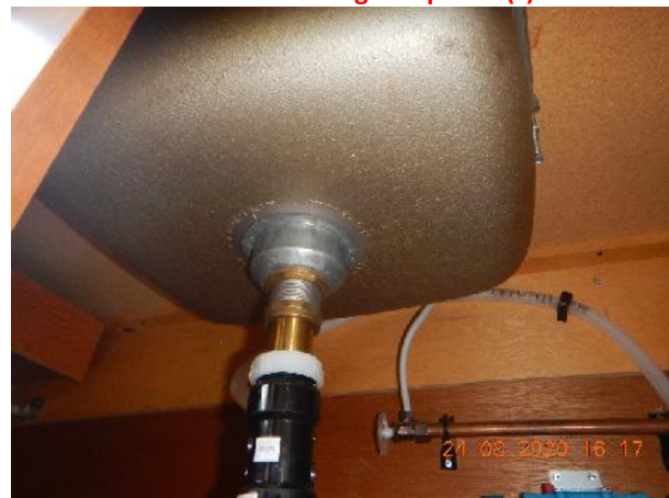
Photo 6 Description: Acoustic sink insulation – Gold Location: 2nd Floor Lunch Room Asbestos: Suspect
