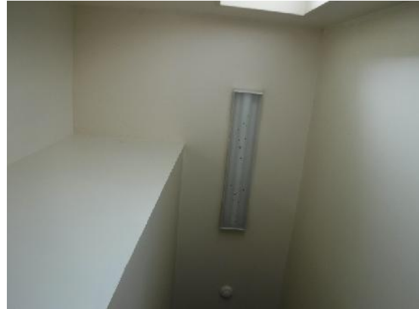
Photo 2 Description: Drywall with joint compound Location: Stairs for Entryway to Mezzanine Asbestos: Suspect
