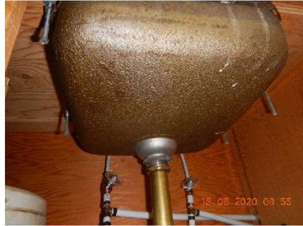
Photo 6 Description: Mastic 2 – Gold/silver Location: Room 1 Asbestos: Suspect
