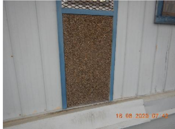
Photo 2 Description: Aggregate panel Location: Exterior Asbestos: Suspect
