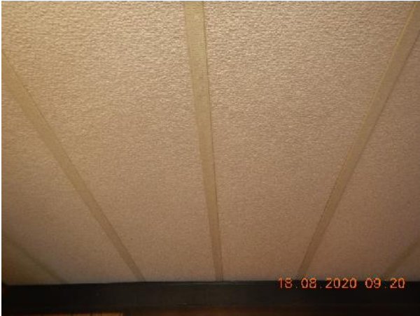
Photo 9 Description: Acoustic ceiling tile 1 – Textured
