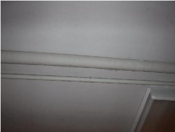
Photo 21 Description: Asbestos cement parging Location: Hallway by Gym Asbestos: 5% Chrysotile Sample(s): 10555-06
