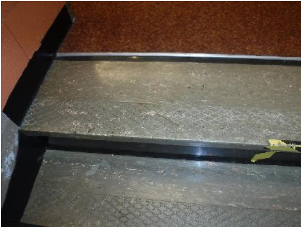
Photo 19 Description: Grey stair tread Location: Mezzanine Accessed by Gym Asbestos: Suspect
