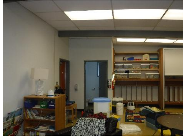
Photo 10 Description: Drywall with joint compound Location: Community Rental B Asbestos: Suspect
