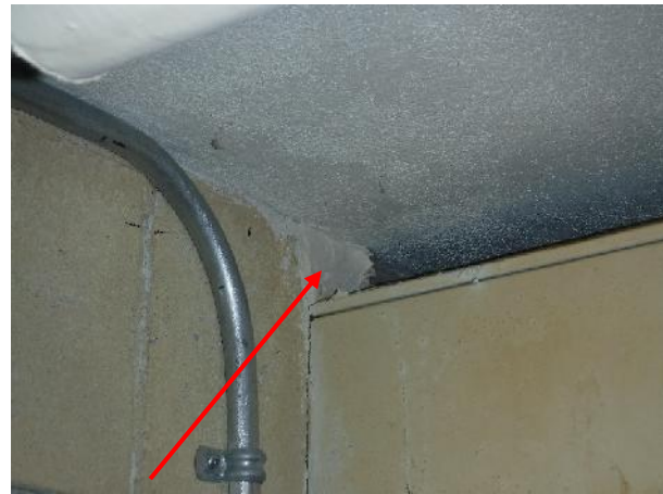
Photo 16 Description: Caulking 2 – White Location: Janitor Room by Gym Asbestos: Suspect
