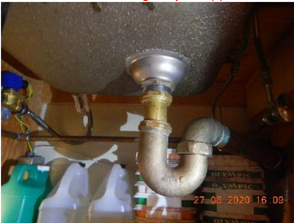
Photo 11 Description: Mastic 1 – Gold/silver Location: Room 105 Asbestos: Suspect
