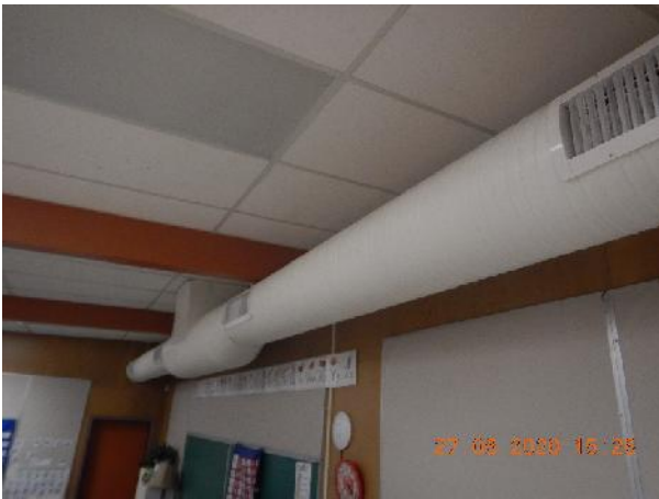
Photo 15 Description: Caulking 1 – Grey (painted white) Location: Room 100 Asbestos: Suspect
