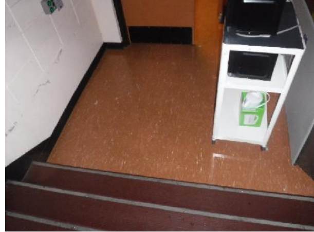
Photo 18 Description: Brown stair tread Location: Hall by Gym Asbestos: Suspect
