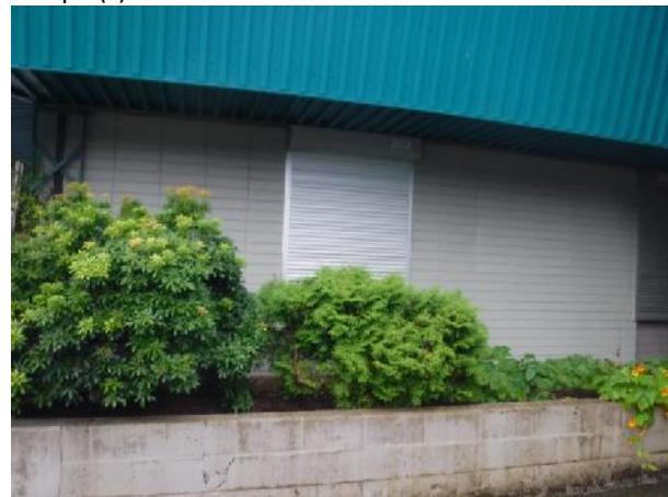
Photo 4 Description: Concrete block Location: Exterior Asbestos: Suspect in cavity
