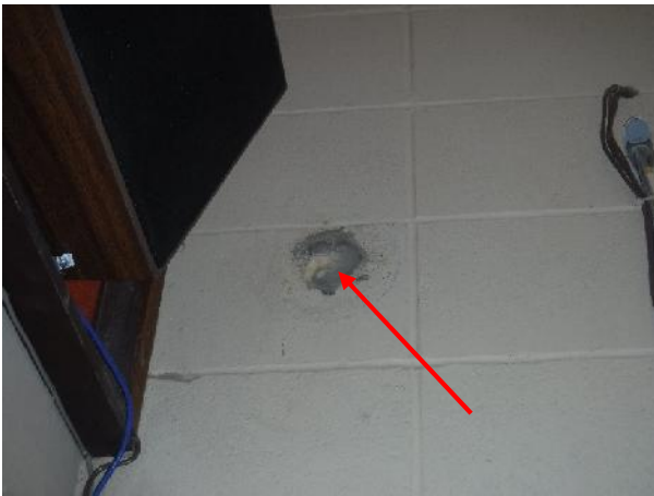
Photo 11 Description: Caulking type 2 – Grey/white Location: Gym Asbestos: Suspect
