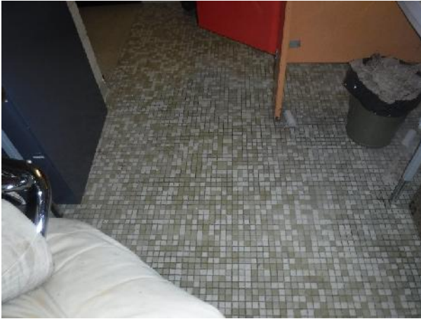
Photo 17 Description: 1/2"x1/2" ceramic tile grout and thinset Location: Room 311 Asbestos: Suspect
