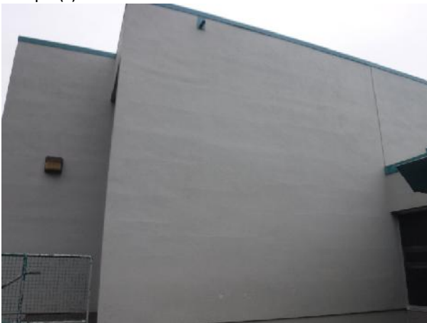
Photo 3 Description: Stucco Location: Exterior Asbestos: Suspect
