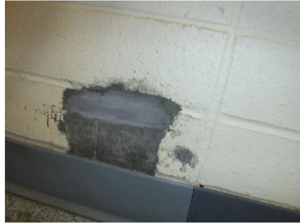
Photo 18 Description: Grey parging Location: Room 208 Asbestos: Suspect
