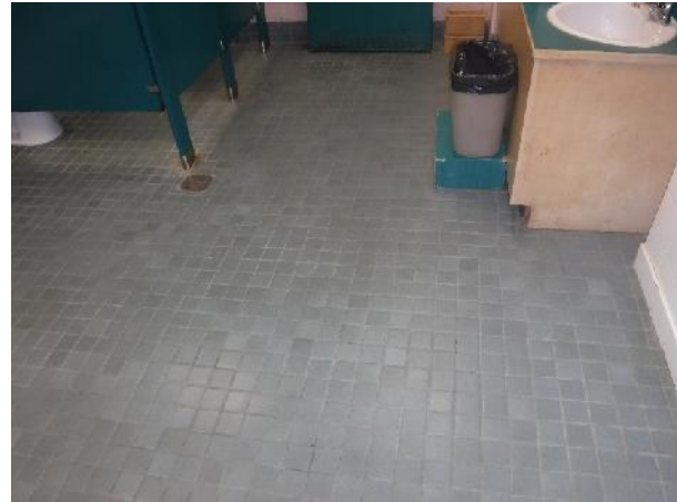
Photo 16 Description: Green 2"x2" ceramic tile grout and thinset Location: Room 209 Asbestos: Suspect
