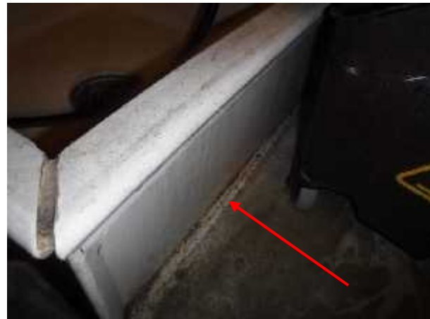
Photo 12 Description: Caulking – White
