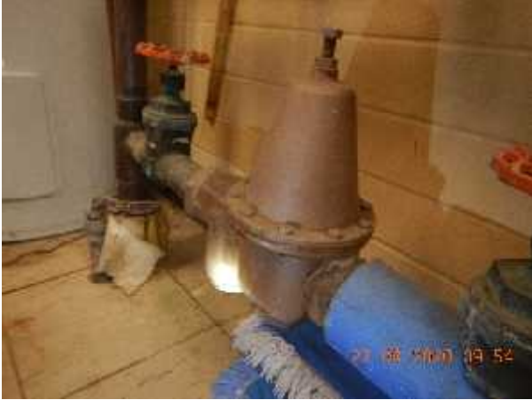
Photo 5 Description: Gasket Location: Janitor's Room Asbestos: Suspect
