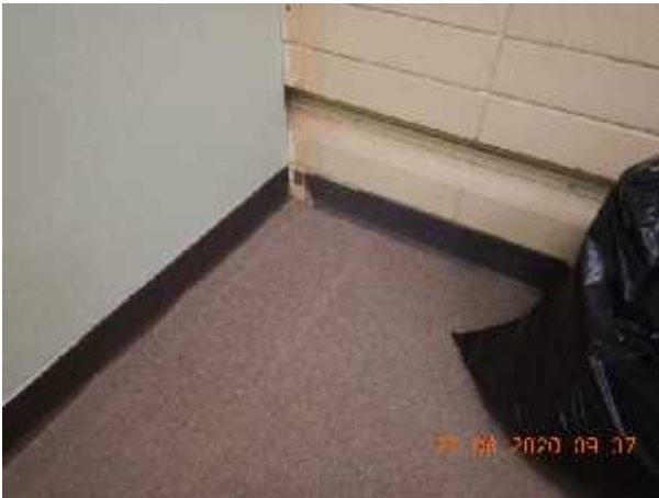
Photo 5 Description: Baseboard adhesive Location: Office A Asbestos: Suspect
