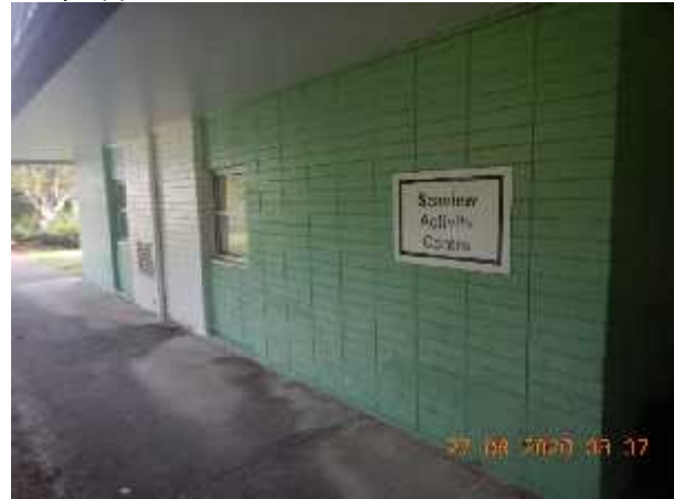
Photo 4 Description: Concrete black (may contain vermiculite) Location: Exterior Asbestos: Suspect
