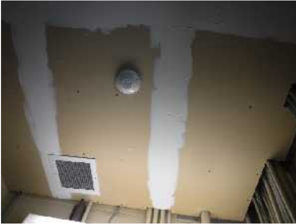
Photo 5 Description: Drywall with joint compound Location: Electrical Room Asbestos: Suspect
