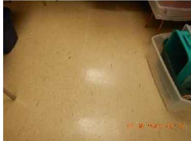
Photo 2 Description: Floor tile 1 – Beige 12"x12" with white/black smear Location: Staff Room Asbestos: 2.3% Chrysotile Sample(s): 30710-2
