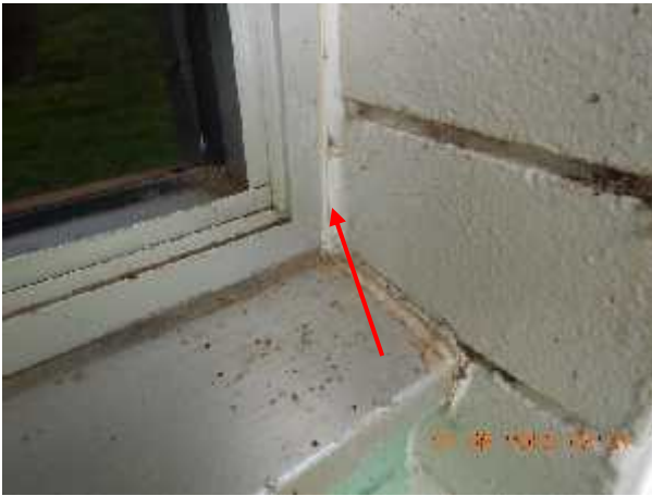
Photo 5 Description: Caulking type 2 – White Location: Exterior Asbestos: Suspect
