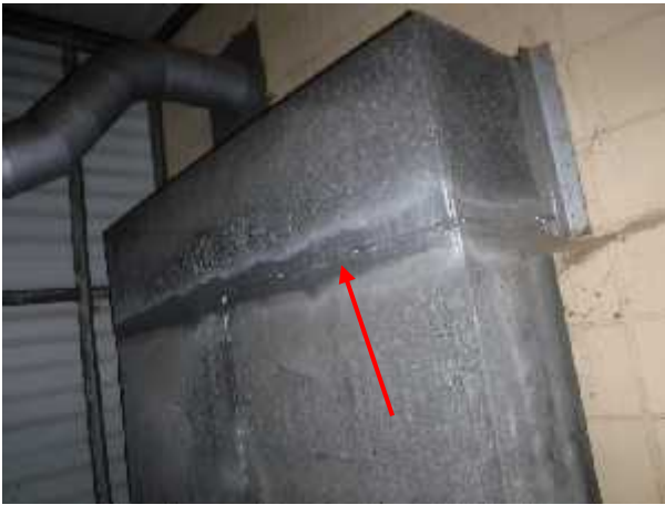
Photo 7 Description: Mastic – Grey Location: Dust Collection Room Asbestos: Suspect
