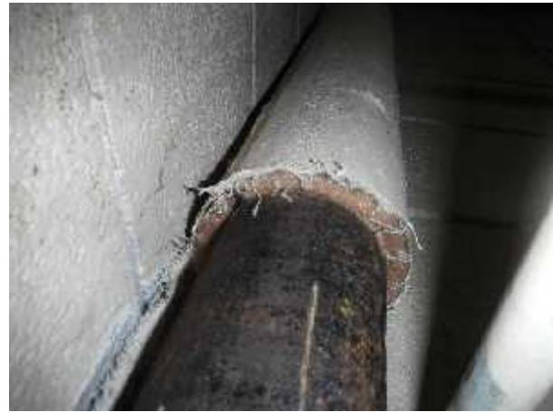
Photo 8 Description: Texture wrapped fibreglass insulation Location: Welding Room Asbestos: Suspect
