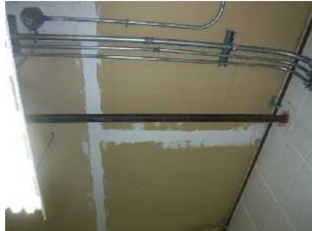
Photo 4 Description: Drywall with joint compound Location: Boiler Room Asbestos: Suspect
