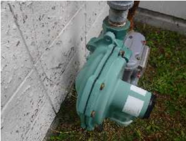
Photo 3 Description: Gasket 2 Location: Exterior Asbestos: Suspect
