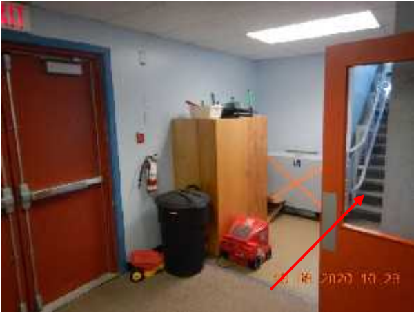
Photo 21 Description: Stair tread – Marbled grey Location: 9-12 Wing Stairway to Basement Asbestos: Suspect
