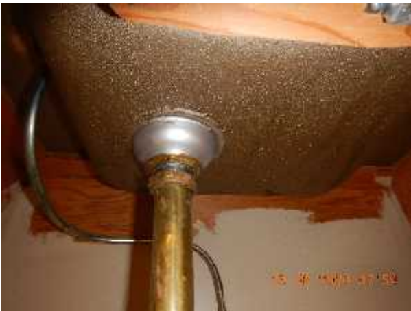
Photo 19 Description: Mastic 2 – Gold Location: Classroom 7 Asbestos: Suspect
