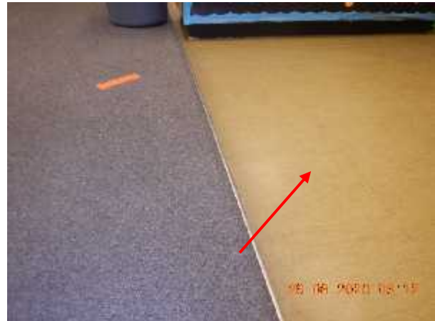
Photo 2 Description: Sheet flooring 2 – Beige and grey streaks Location: Classroom 3 Asbestos: 2.9% Chrysotile Sample(s): 30010-1
