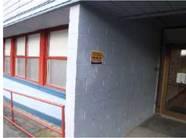
Photo 10 Description: Concrete block wall Location: Exterior Asbestos: Suspect
