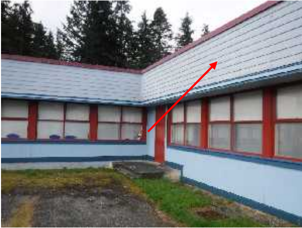
Photo 9 Description: Cement board Location: Exterior Asbestos: Suspect
