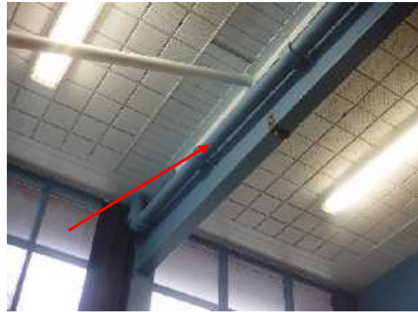
Photo 24 Description: Cement pipe – Painted blue Location: Gym Asbestos: Suspect
