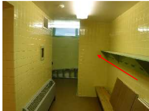
Photo 12 Description: Ceramic tile 1 – 4"x4" beige Location: Men's Washroom Asbestos: Suspect concealed asbestos leveling compound(s)
