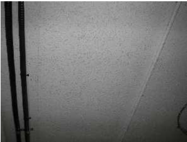
Photo 11 Description: Texture coat Location: Electrical Room Asbestos: Suspect
