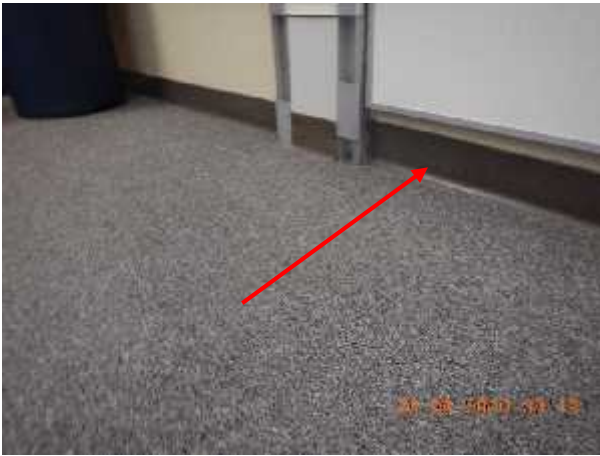
Photo 27 Description: Baseboard adhesive Location: Classroom 3 Asbestos: Suspect
