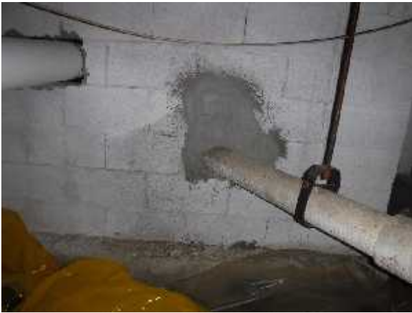
Photo 23 Description: Parging – Grey Location: Crawl Space Asbestos: Suspect
