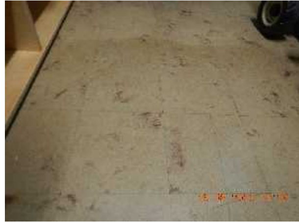
Photo 14 Description: Floor tile 3 – Beige with red streaks Location: Gym Storage Asbestos: Suspect
