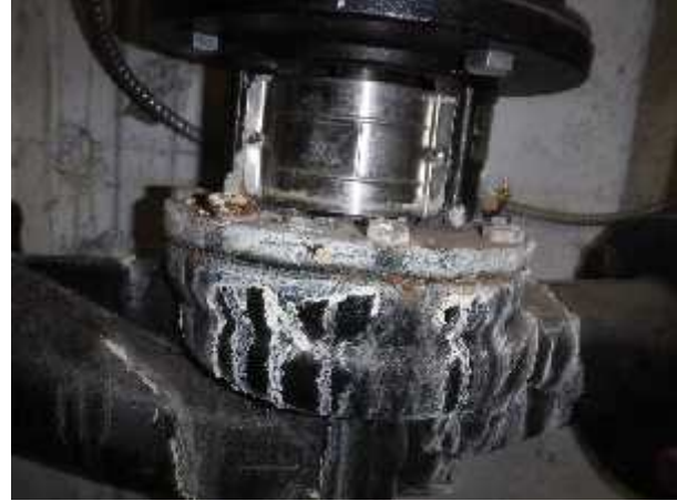
Photo 26 Description: Pipe gaskets Location: Boiler/Hot Water Room Asbestos: Suspect
