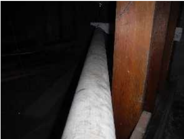
Photo 7 Description: Cement pipe Location: Crawl Space Asbestos: 15% Chrysotile Sample(s): 30010-17
