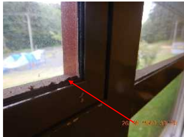
Photo 20 Description: Window putty 1 – Black Location: Classroom 11 Asbestos: Suspect
