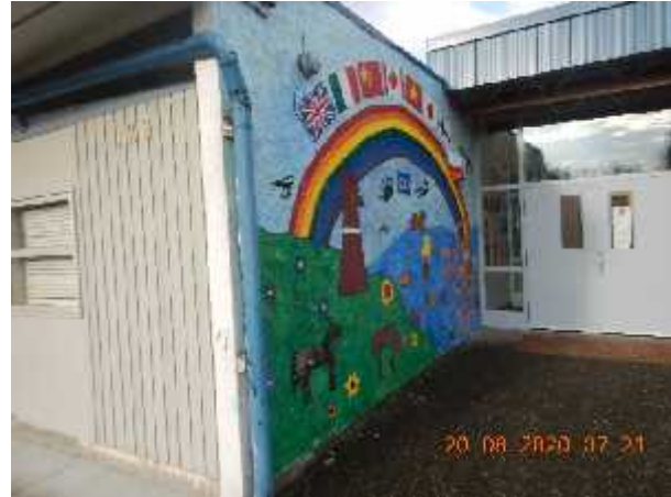
Photo 6 Description: Stucco Location: Exterior Asbestos: Suspect
