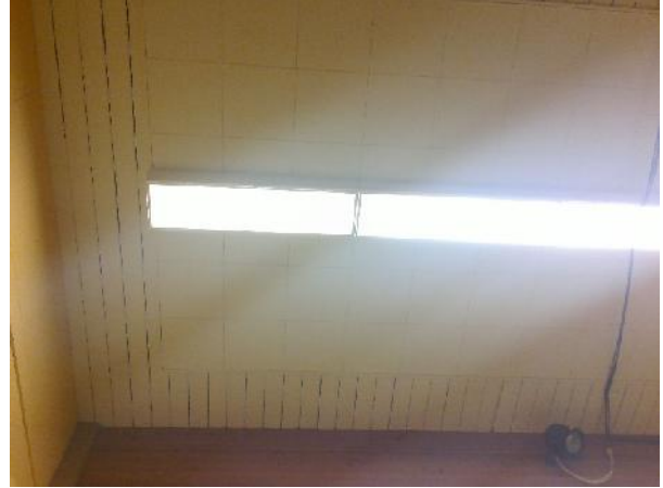
Photo 6 Description: Fluorescent light tubes Location: Gymnasium Lead: Tubes contain mercury, ballasts may contain PCBs Sample(s): None
