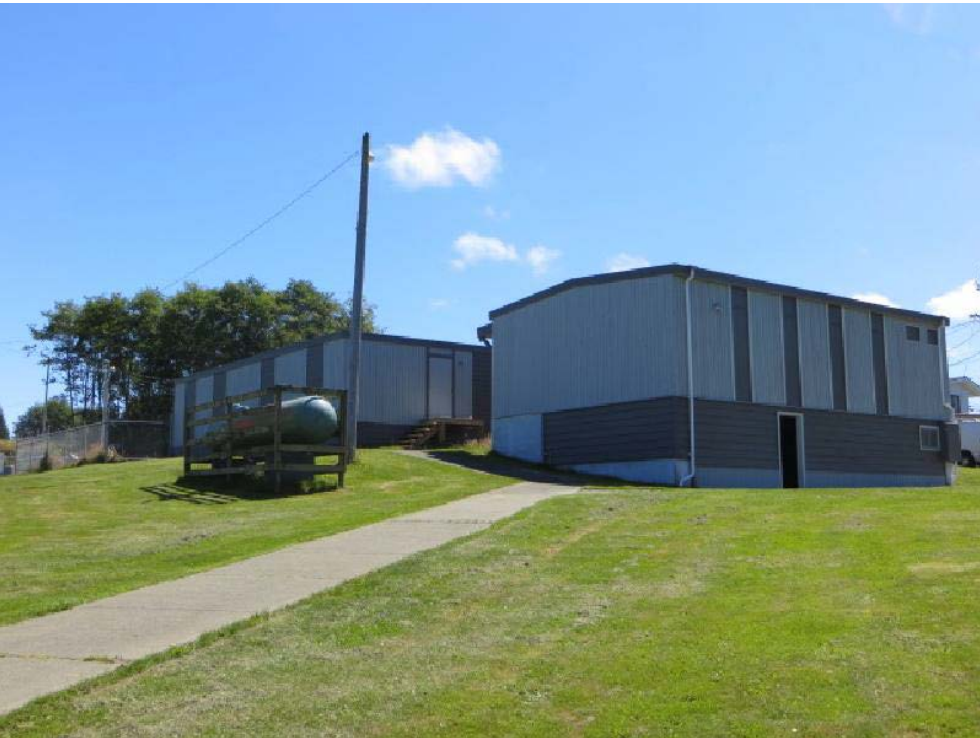
Maintenance Shop 2 – south
