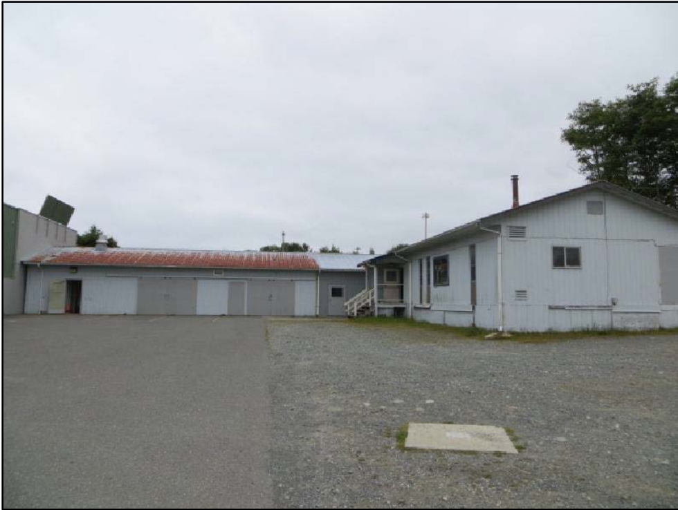
Maintenance Shop 1 – south
