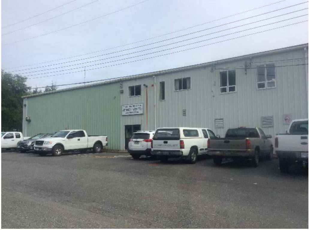
Maintenance Shops – old Tacan site
