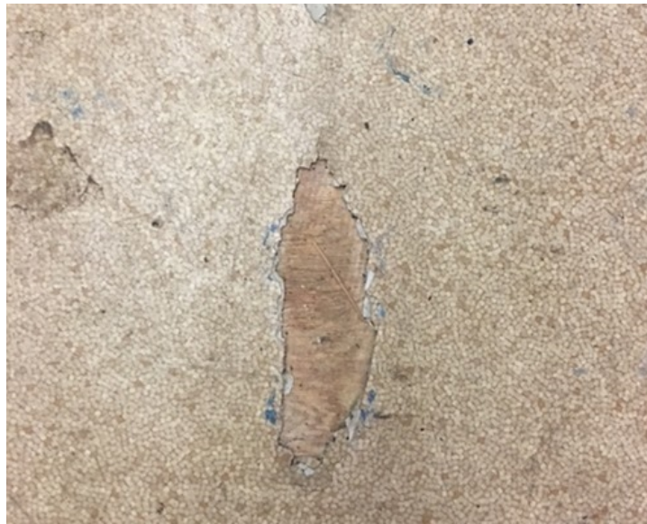
Sheet Flooring - SF2-Small Beige Mosaic (contains 30% Chrysotile asbestos)
