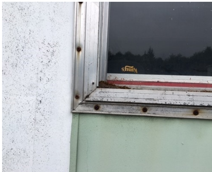
Caulking - Off White (contains 15% Chrysotile asbestos)
