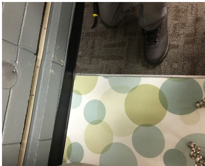
Sheet Flooring - Flooring below with Circles Pattern (contains 15% Chrysotile asbestos)
