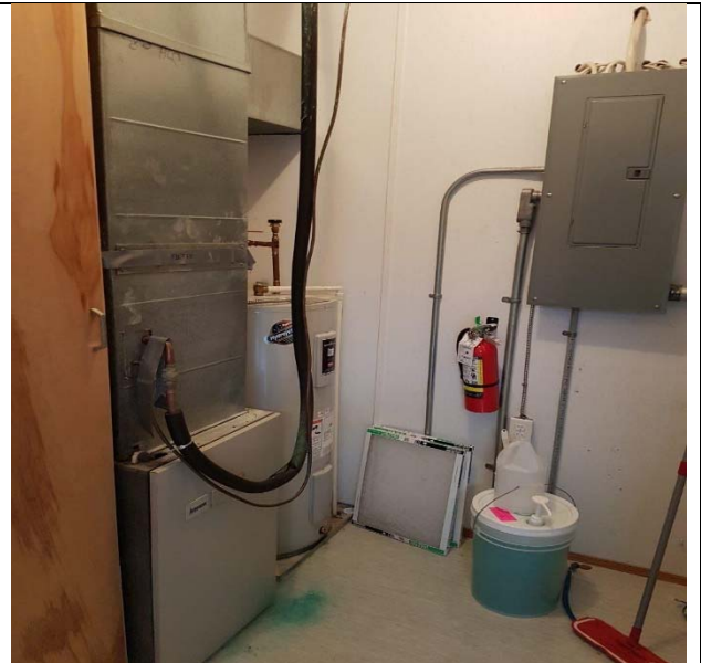
Photo: 33310-6 Location: Furnace Room Description: Sheet Flooring Asbestos: No Asbestos Detected
